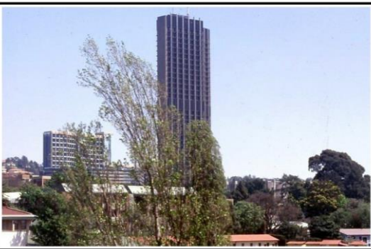
Fig.156-2333. Garden Court Milpark Hotel in Johannesburg City (Left Building).
